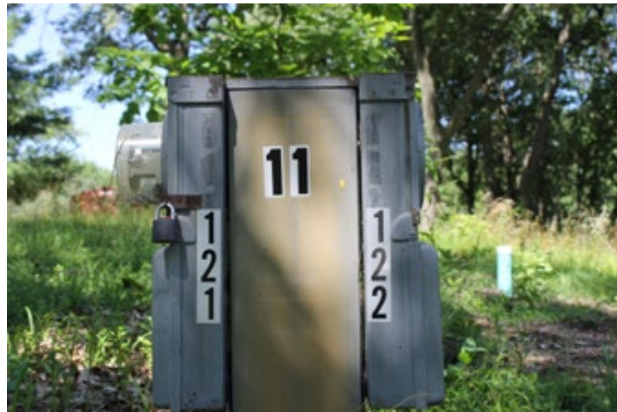
Here is the pedestal with the refreshed numbers and the Section identified in the middle. The section numbers are 3-inch vinyl reflective and the lot numbers are 2-inch vinyl reflective. These were purchased at Woody's True Value Hardware Store.
